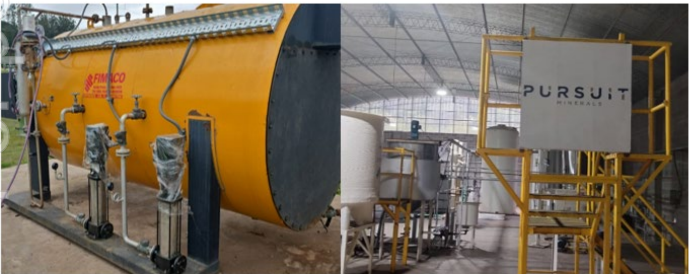
Figure 4: Boiler installation at the 250tpa Lithium Carbonate Plant in Salta.
