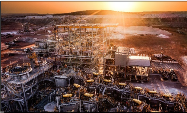
Figure 4: Aerial view of the process plant
