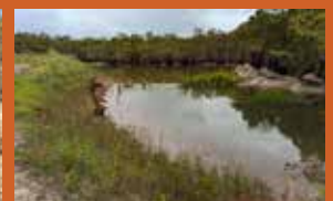
Namaleta Creek Realignment – January 2025
