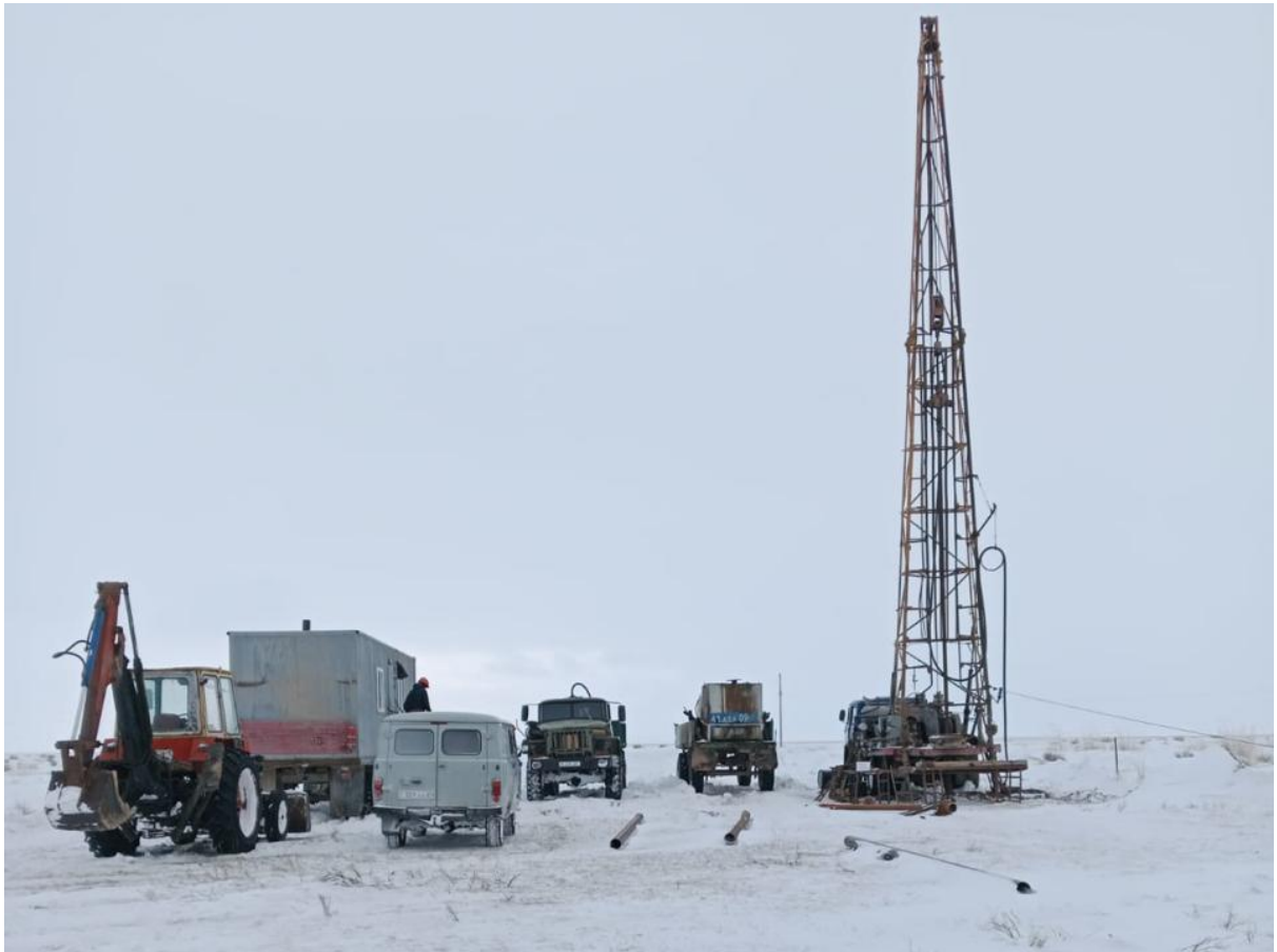
Figure 4 – Water bore drilling underway in the Sherubainura River Aquifer
