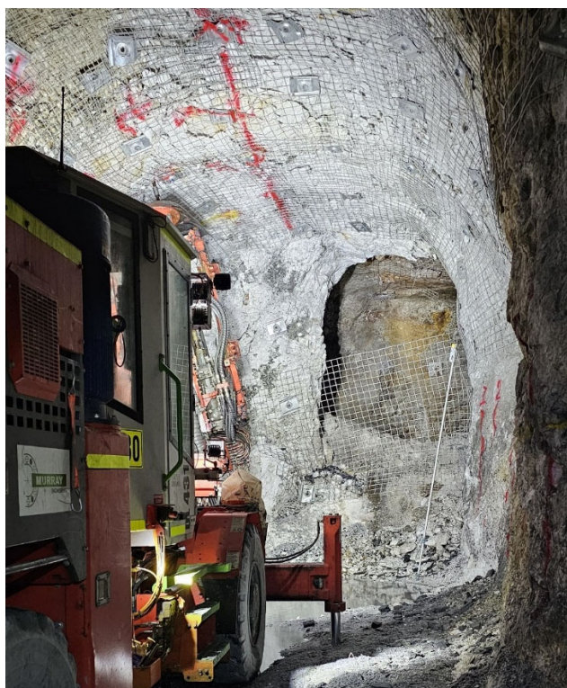
Figure 3: Longhole drill in action, late March 2025.
