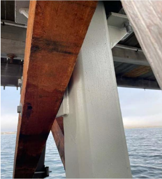
Figure 1: Trial inspection photos showing coatings performing well at the Streaky Bay Jetty, South Australia (April 2025)
