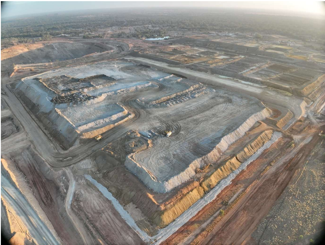
Figure 3: Progressive mine rehabilitation of old heap leach pads underway using clean waste rock from Murrawombie Pit
