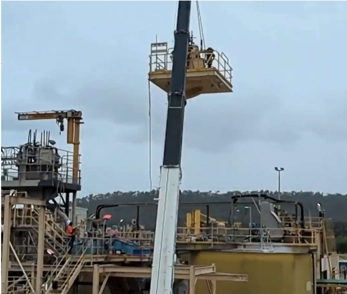
Figure 5: Secondary cyclone circuit being installed
