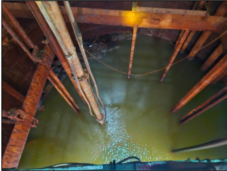
Photo 4: Mine Dewatering 500m 3 /hr (proof of concept).
