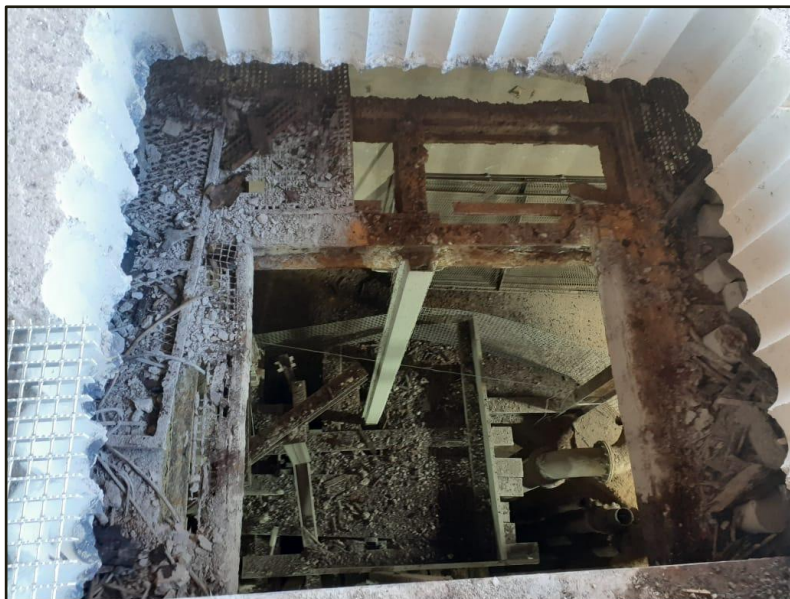
Photo 3: Hutchings Shaft Cement Slab Opened.
