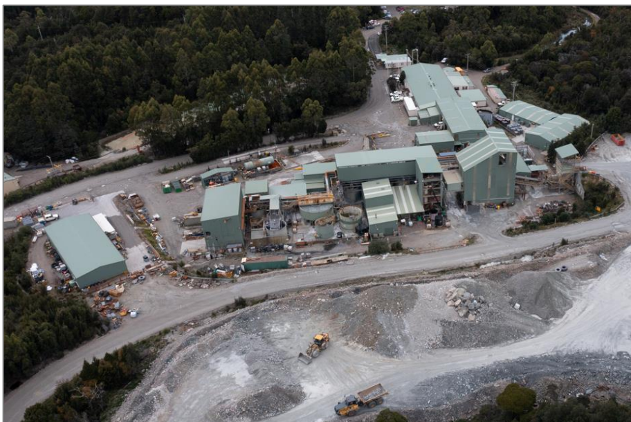
Figure 1 - Henty 300ktpa CIL Plant & Administration Complex
