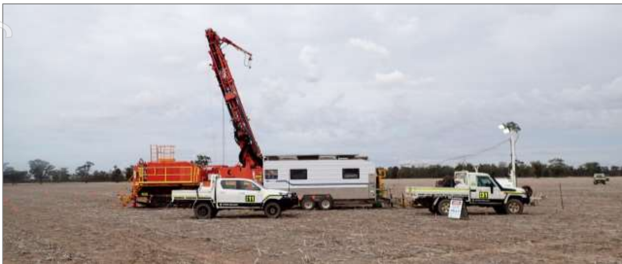
Figure 1. Drilling rig on site at Calais
