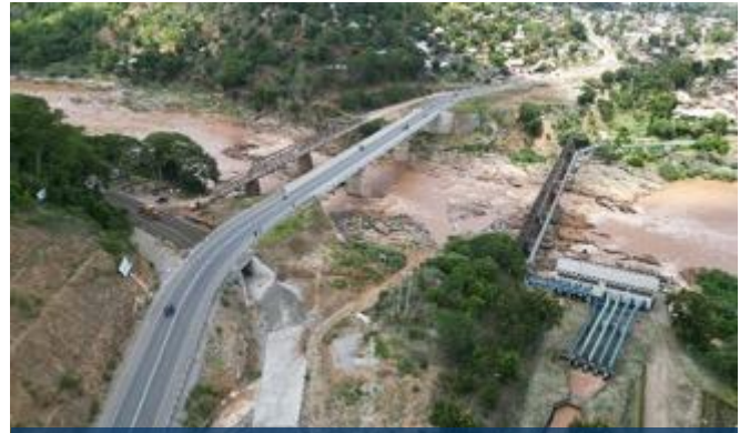
Great Ruaha Bridge
