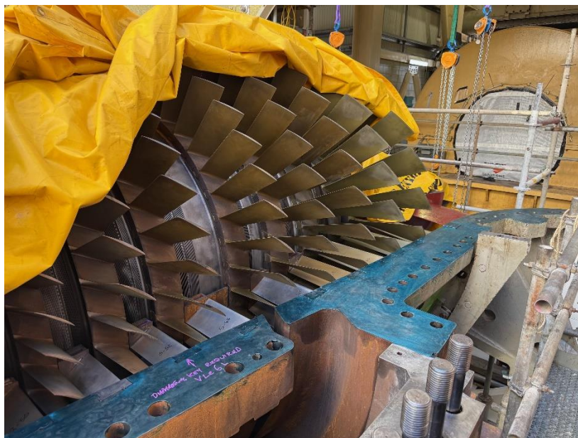
Image: Overhaul compressor stages of TPS turbine
