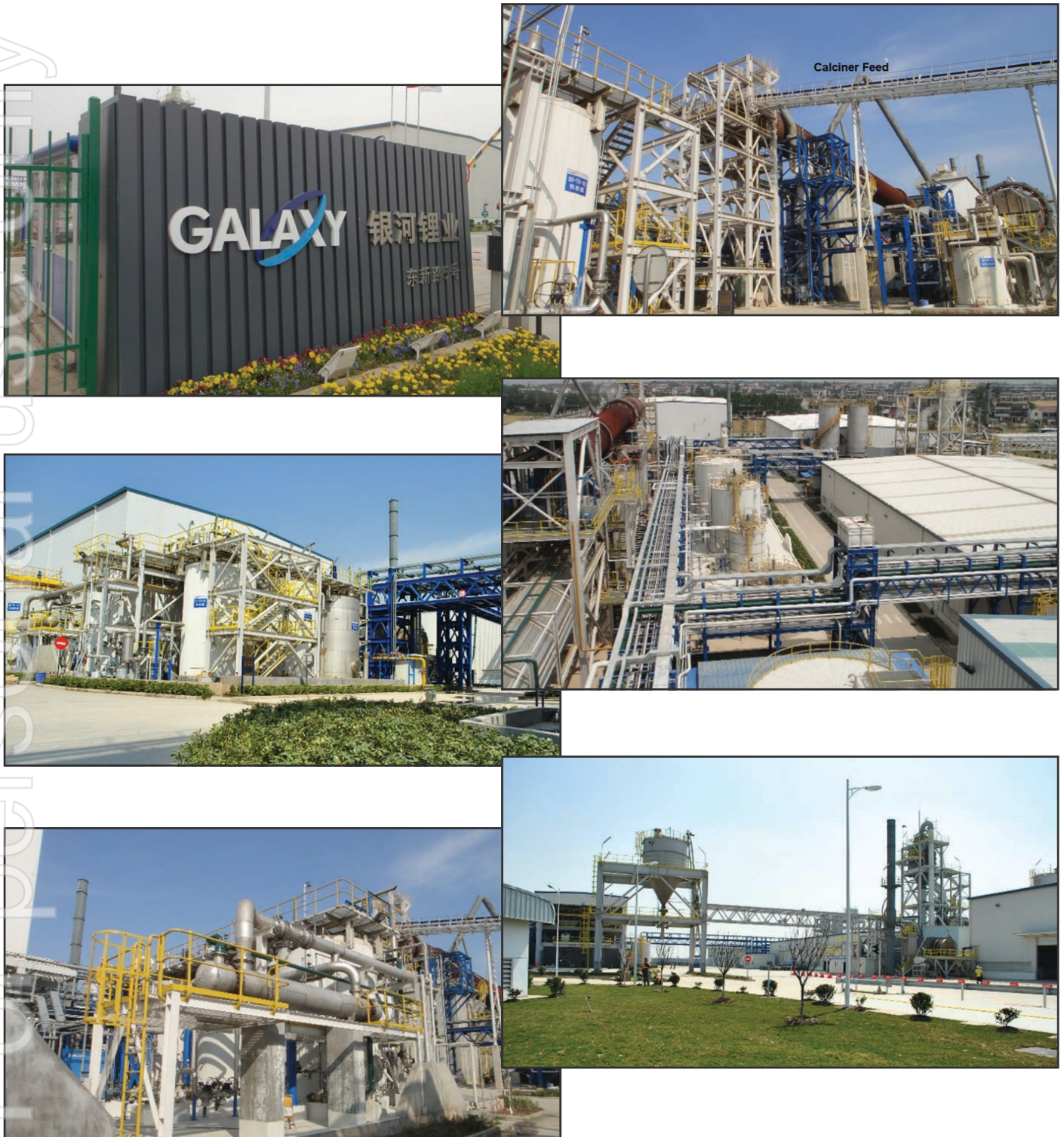
Figure 6: Galaxy Jiangsu Lithium Carbonate Plant
