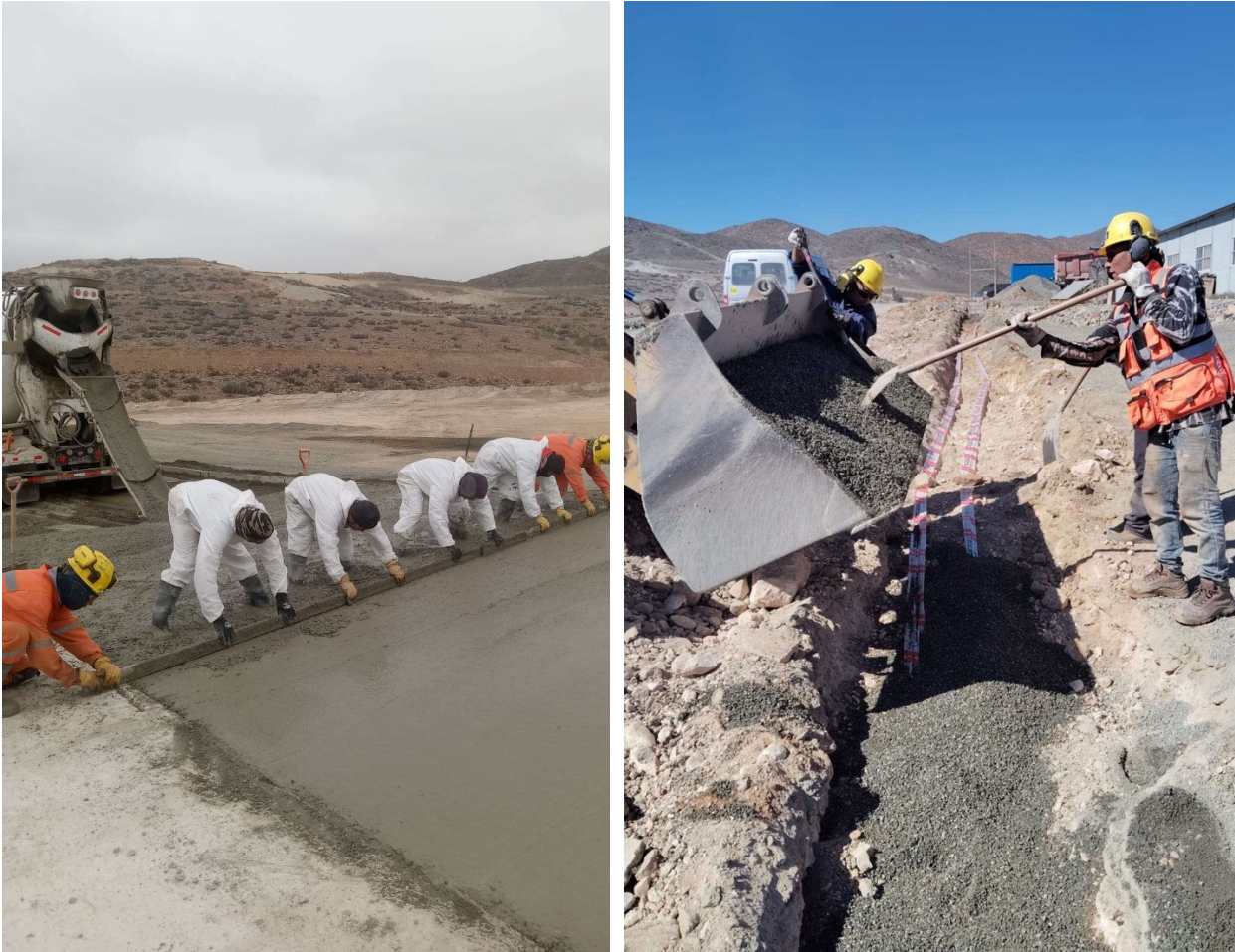
Figure 2: Construction activities at Mariposa Mine
