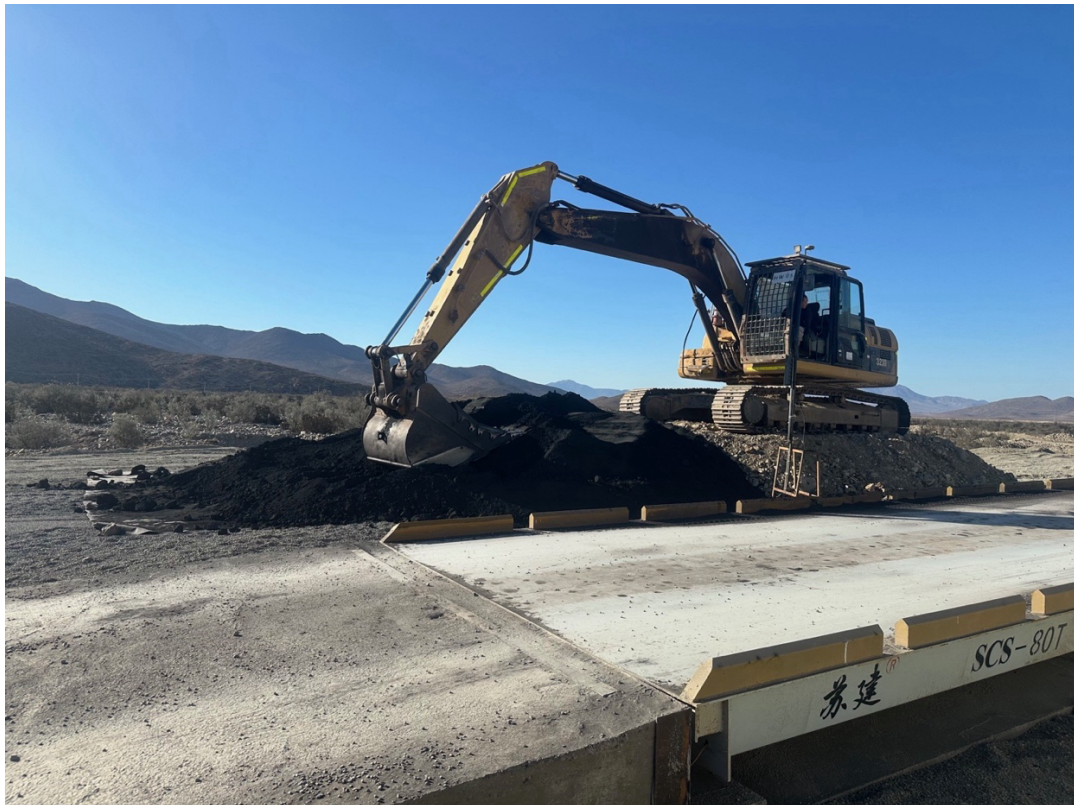
Figure 3: Ore loading at Mariposa Mine
