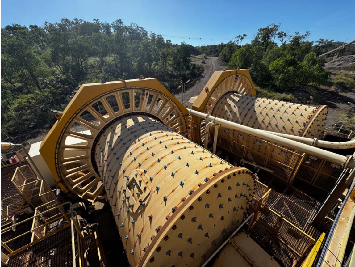
Ball Mill (foreground) and Sag Mill at Mungana
