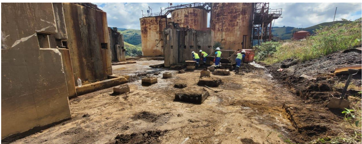
Figure 1: Cleaning of old mill structures in preparation for drilling and blasting
