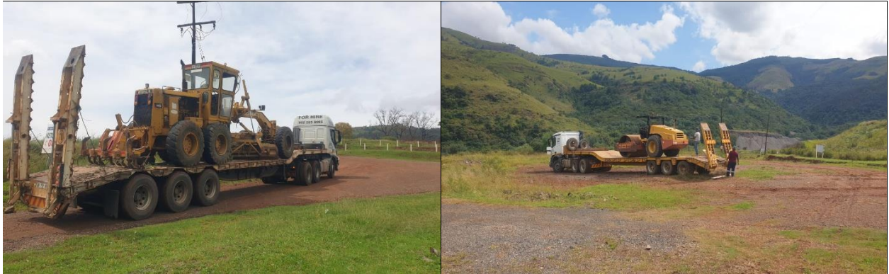
Figure 2: Delivery of contracted Grader and Roller
