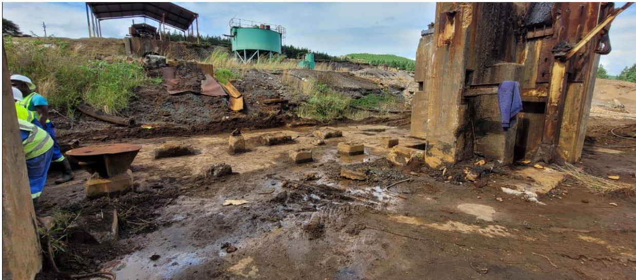
Figure 6: Old mill civils to be removed
