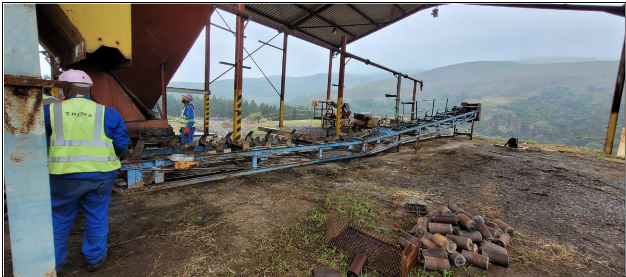
Figure 5: Removal of old conveyor belt structure
