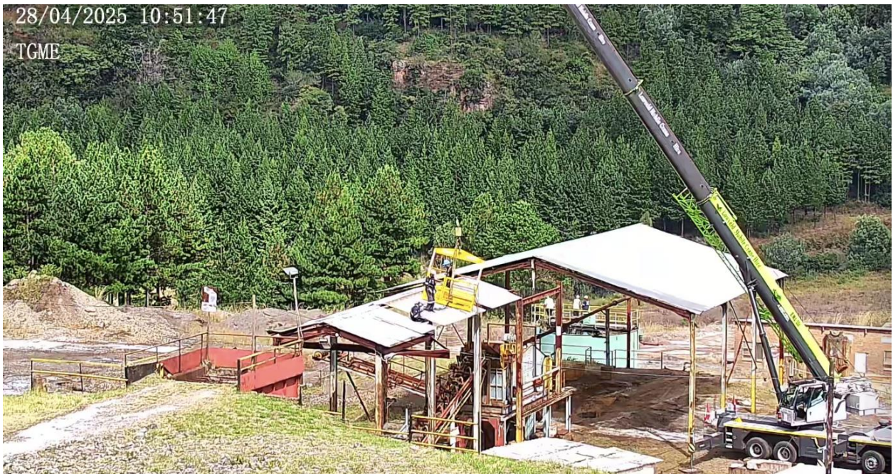
Figure 3: Removal of old mill sections
