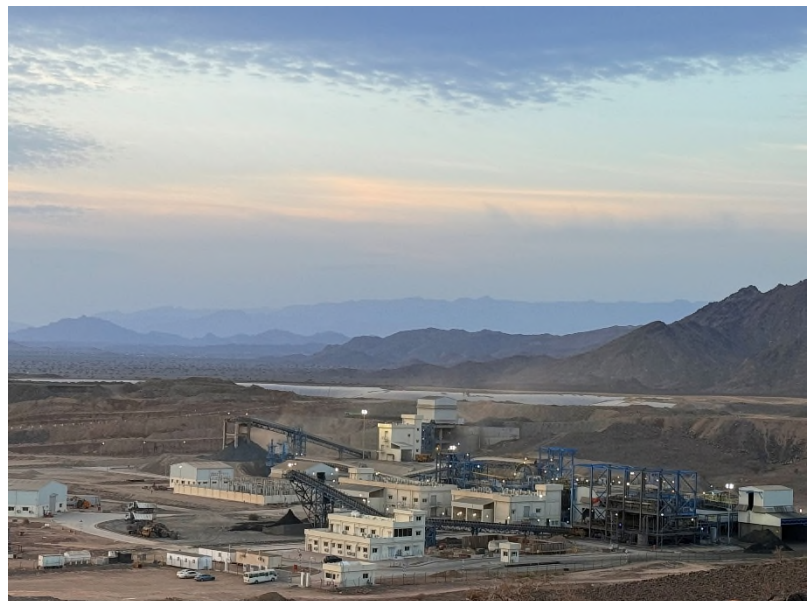
Image: Wash-hi copper-gold processing plant
