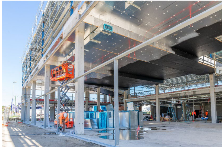
Image 4. Dealership fitout progress
