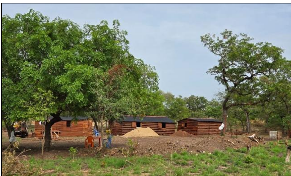
Figure 5 – Low cost and environmentally friendly exploration camp set up at the Dadjan Gold Project.
