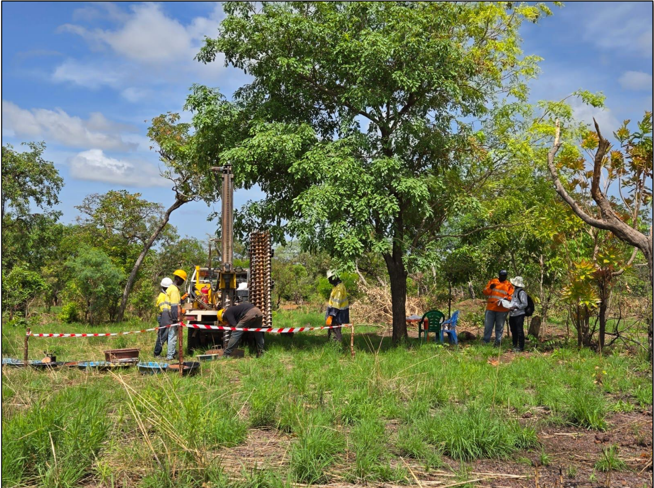
Figure 1 – Power auger drilling underway at the Dadjan Gold Project, located in the Siguiri Basin, Guinea.
