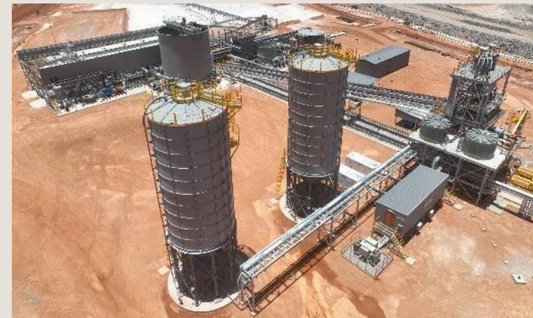
Aerial view of the paste plant, capable of supporting future 4Mtpa operation
