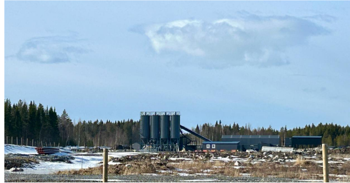
Talga's Anode Refinery site April 2025
