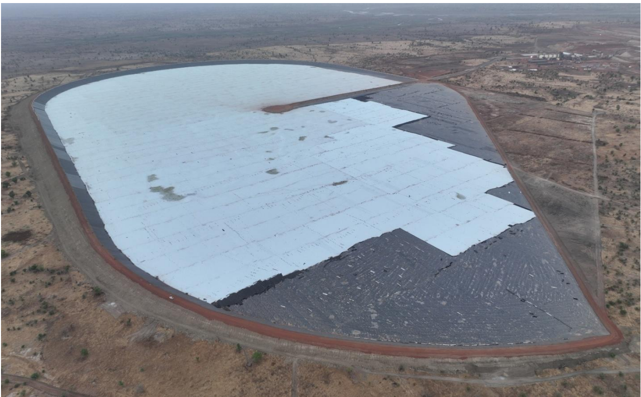
Photo 5: Kiaka tailings storage facility
