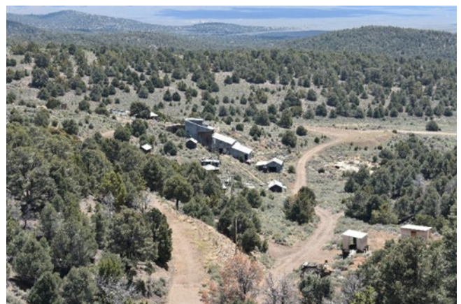
Photo 6. View looking eastwards from the Thomas W Shaft showing the Mill, various workshops and buildings.
