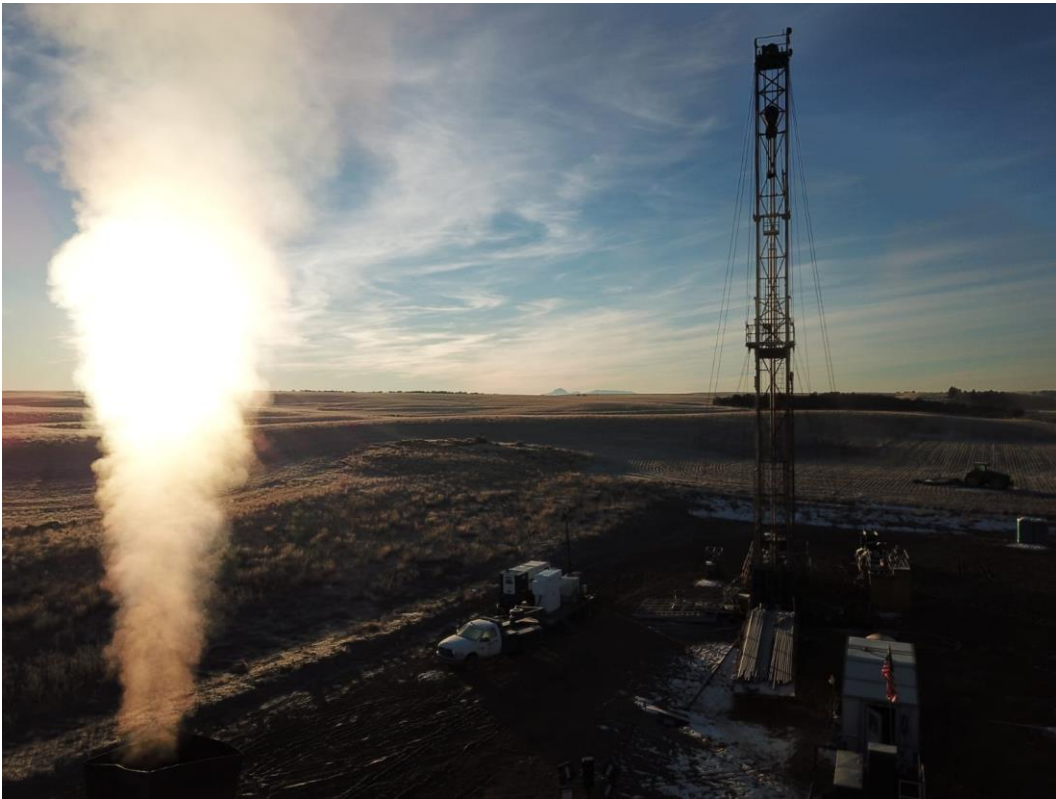
Figure 1: Jesse-1A flare-stack venting reservoir gas and helium to surface during flow-testing in December 2023
