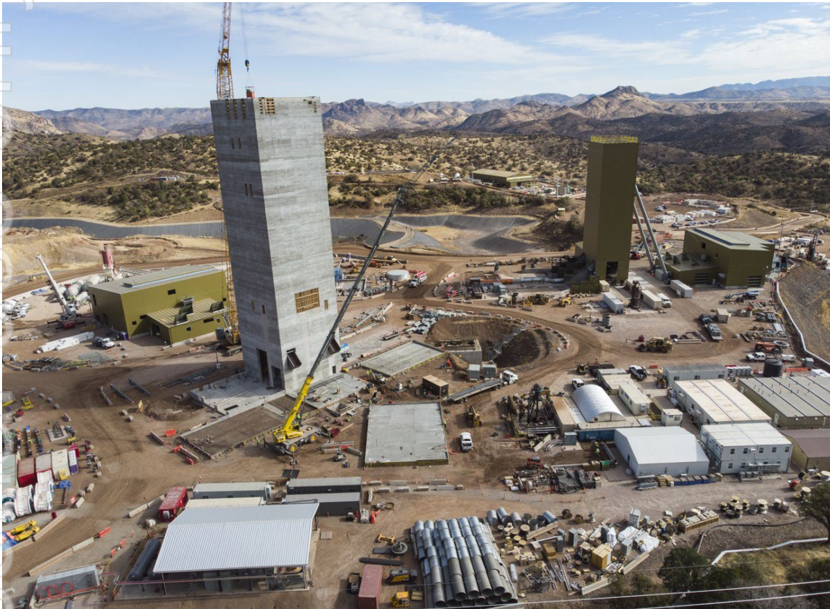
Construction of main shaft (left), ventilation shaft (right) and tailings storage (rear)
