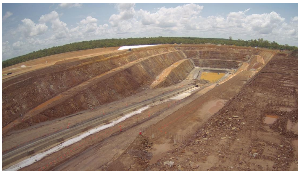
Figure 6-7 BP33 Current Boxcut
