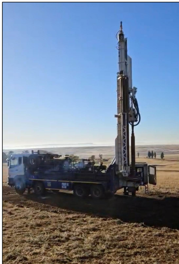
Figure 1: shows drilling rig on site for spudding well 271-KA03PT10
