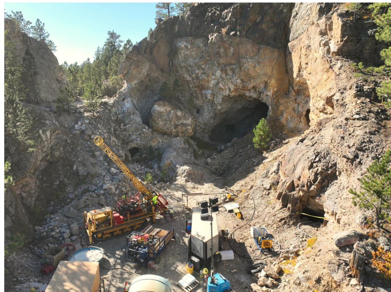
Drilling at the Tin Mountain Project, October 2024
