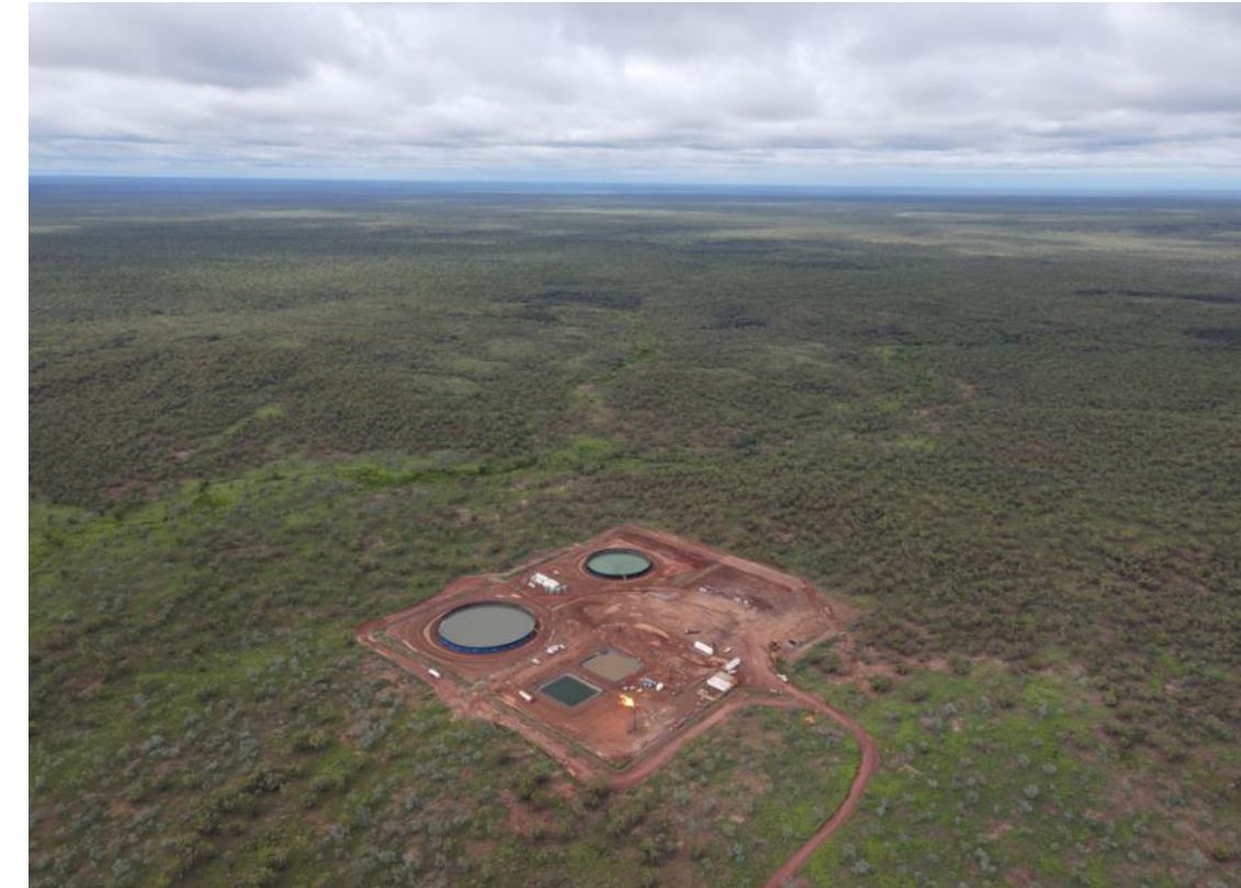
Carpentaria 2H and 3H well pad from above
