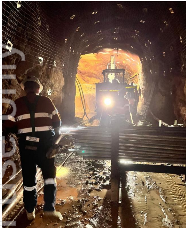
SOZ Underground Mine
