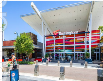
Rockingham Centre 1 Rockingham, WA Regional Shopping Centre
