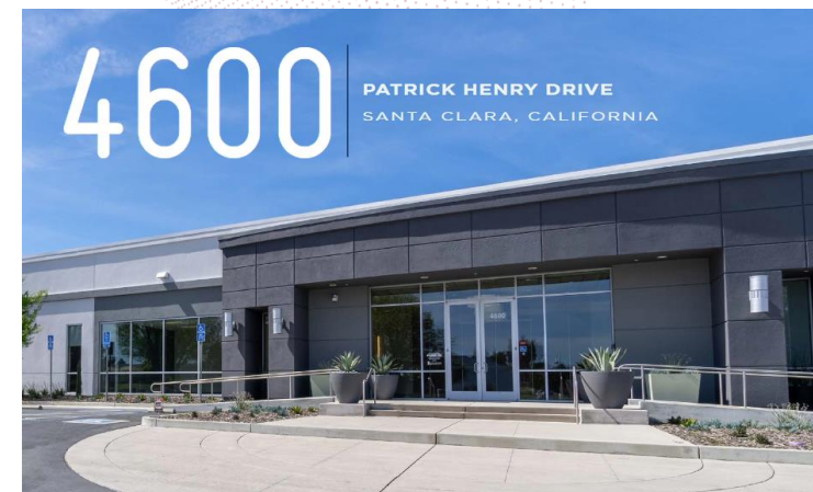
State-of-the-art facility in Santa Clara, California
