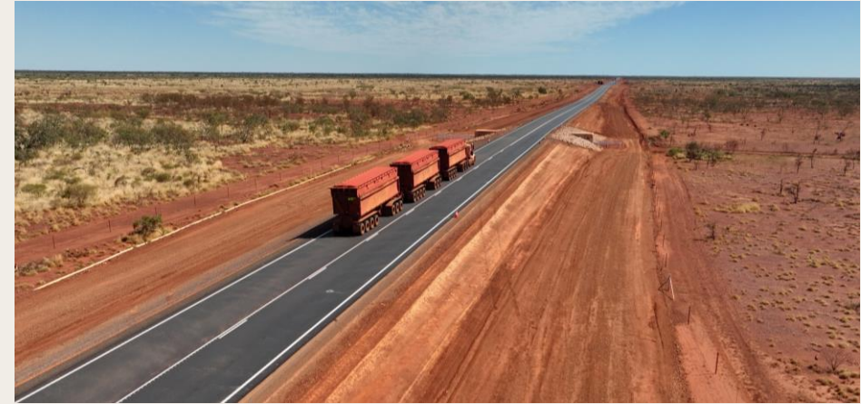
Completed upgrades on MinRes haul road
