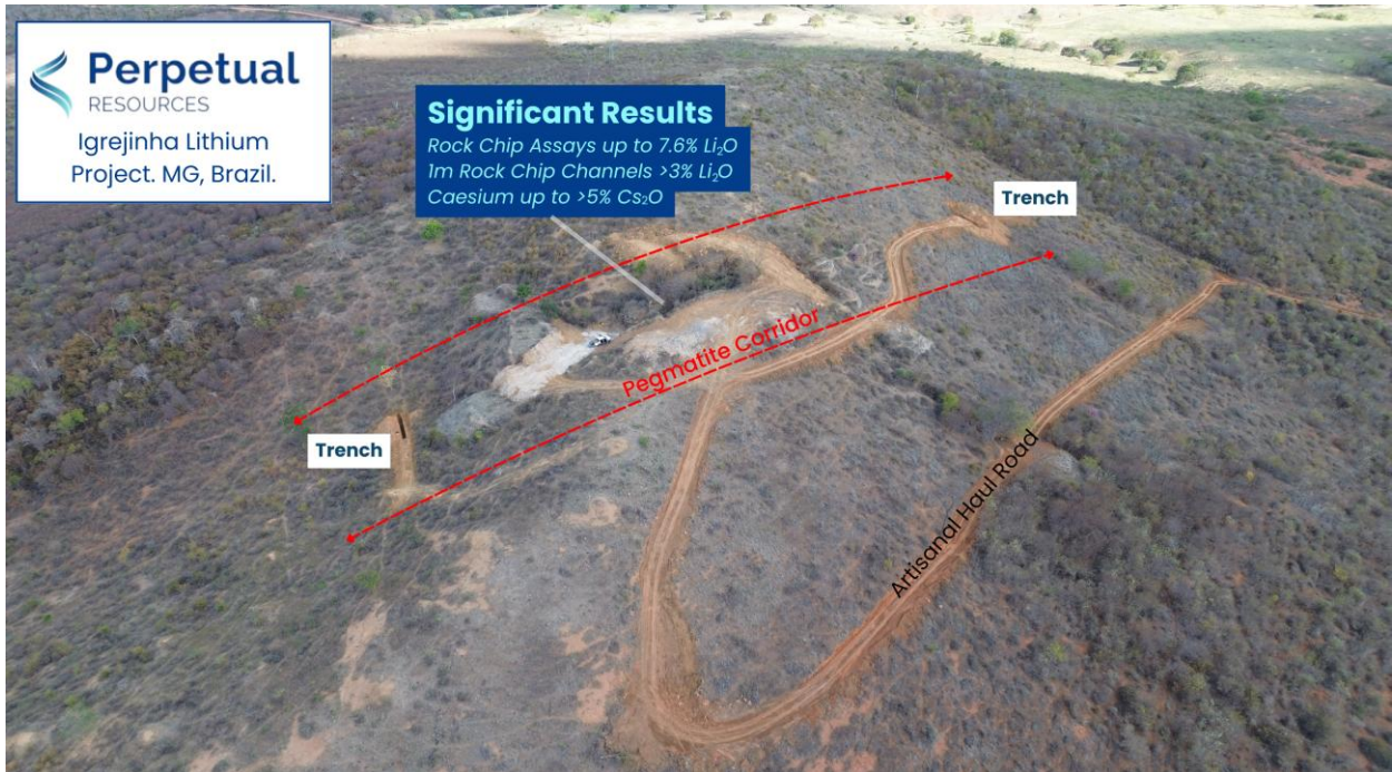
Figure 4 – Access, Trenching and Drilling Preparation at Igrejinha Pegmatite (Licence 830851/2010), for prior results refer ASX announcements on 18 th February, 7 th March & 24 th April 2025.
