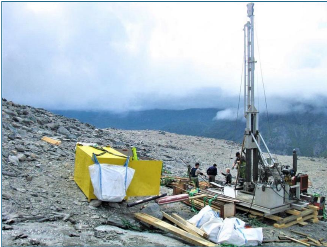
Figure 3 Diamond drilling 2013 over kakortokite surface outcrop (in foreground) at the Fjord deposit
