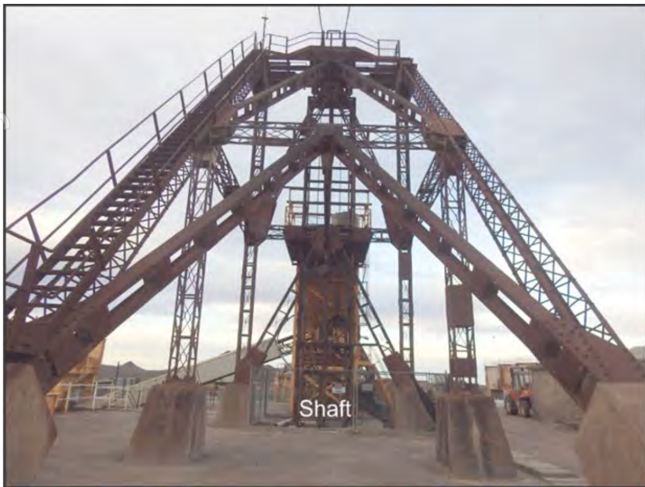
Photo 3-6: Pinnacles Shaft Source: ERM
