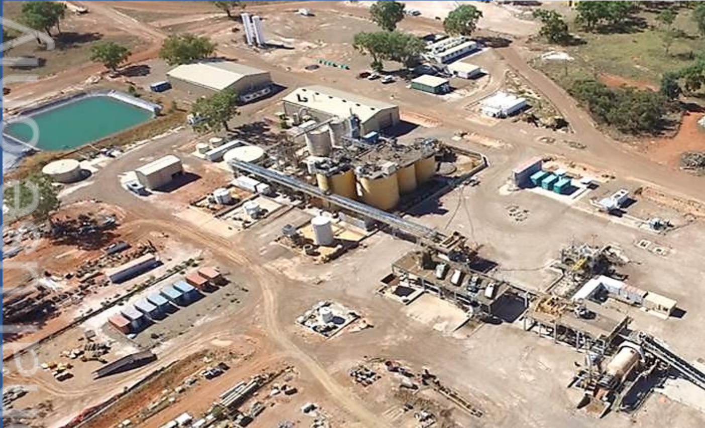
Figure: Aerial view of the existing Wonawinta 1Mtpa Processing Plant showing the Ball Mill (bottom right) and CIL tanks (centre-left).
