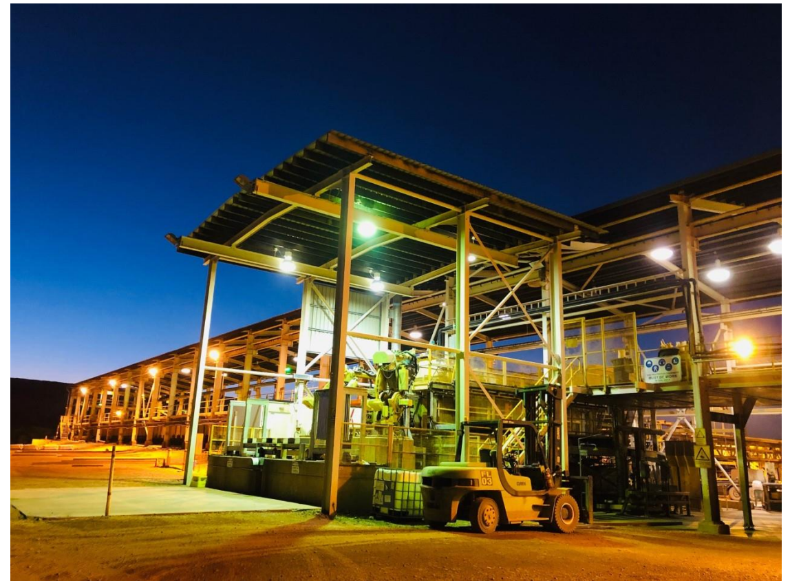
Mount Kelly Copper Processing Facility (Source: Austral Resources)
