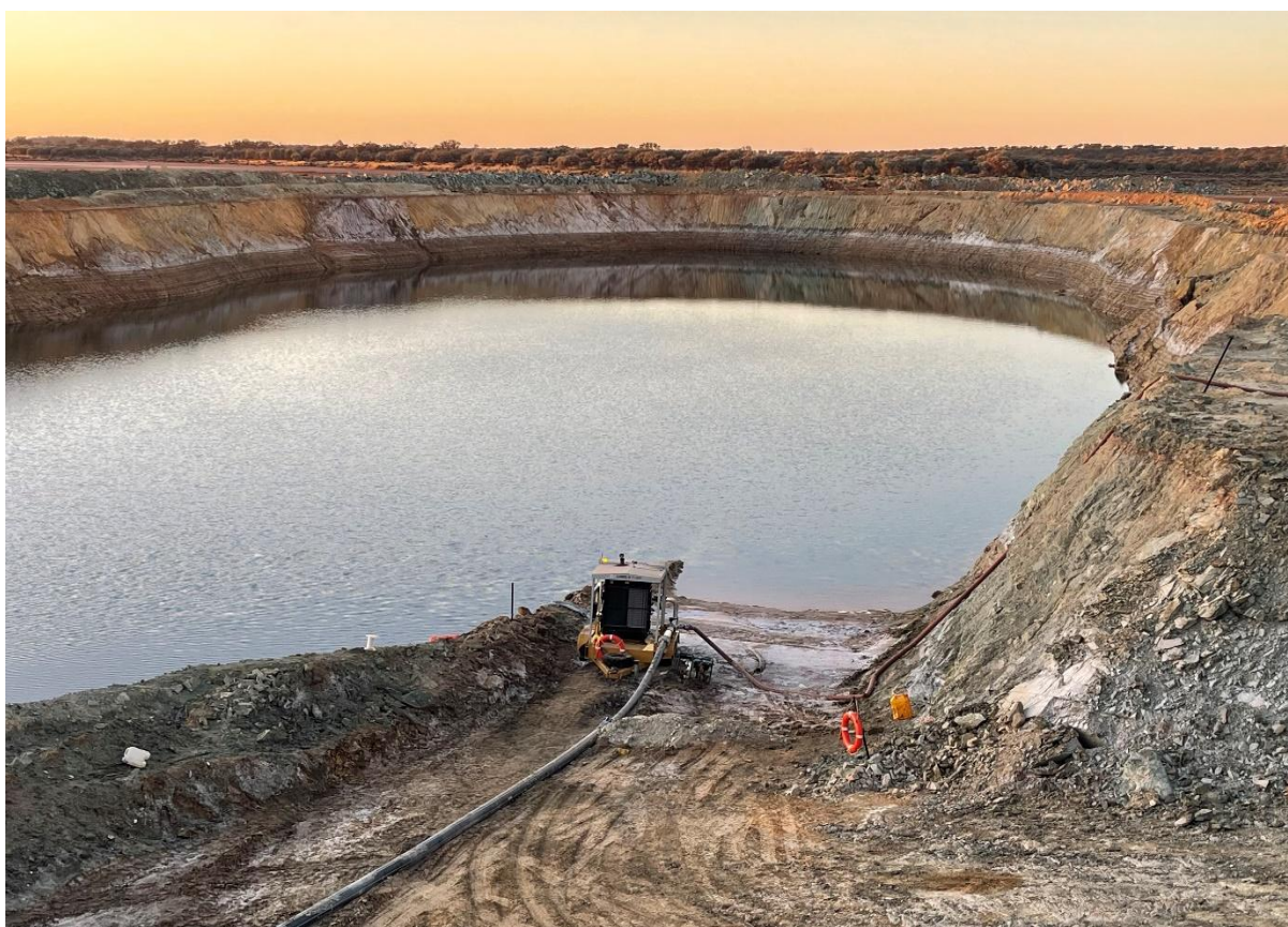
Plates 2 & 3 Progress of Dewatering of the Devon Pit - April 2025 (top) and 25 May 2025 (bottom)
