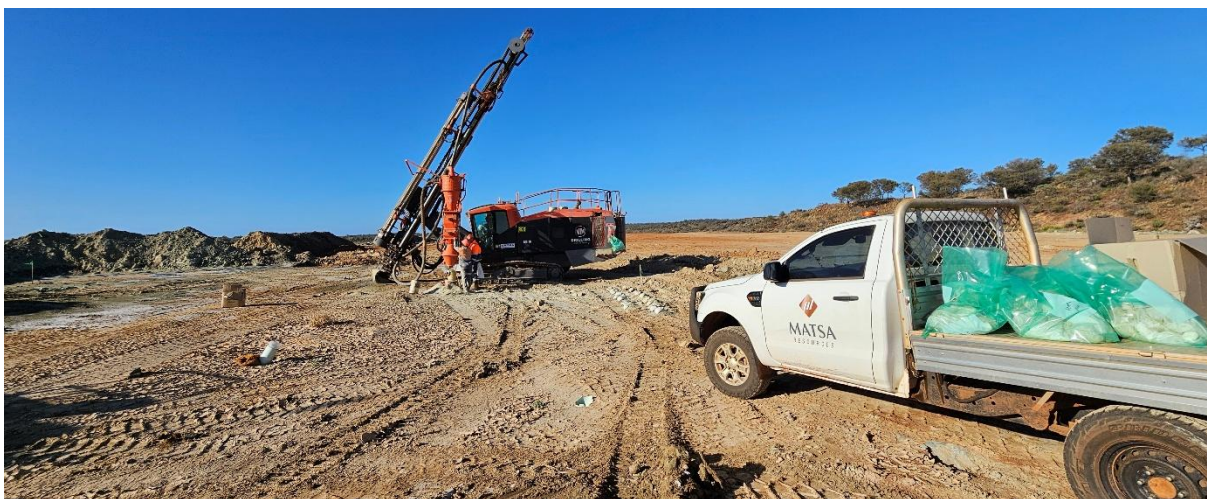
Plate 5 Drill rig is on site to define ore blocks (grade control)
