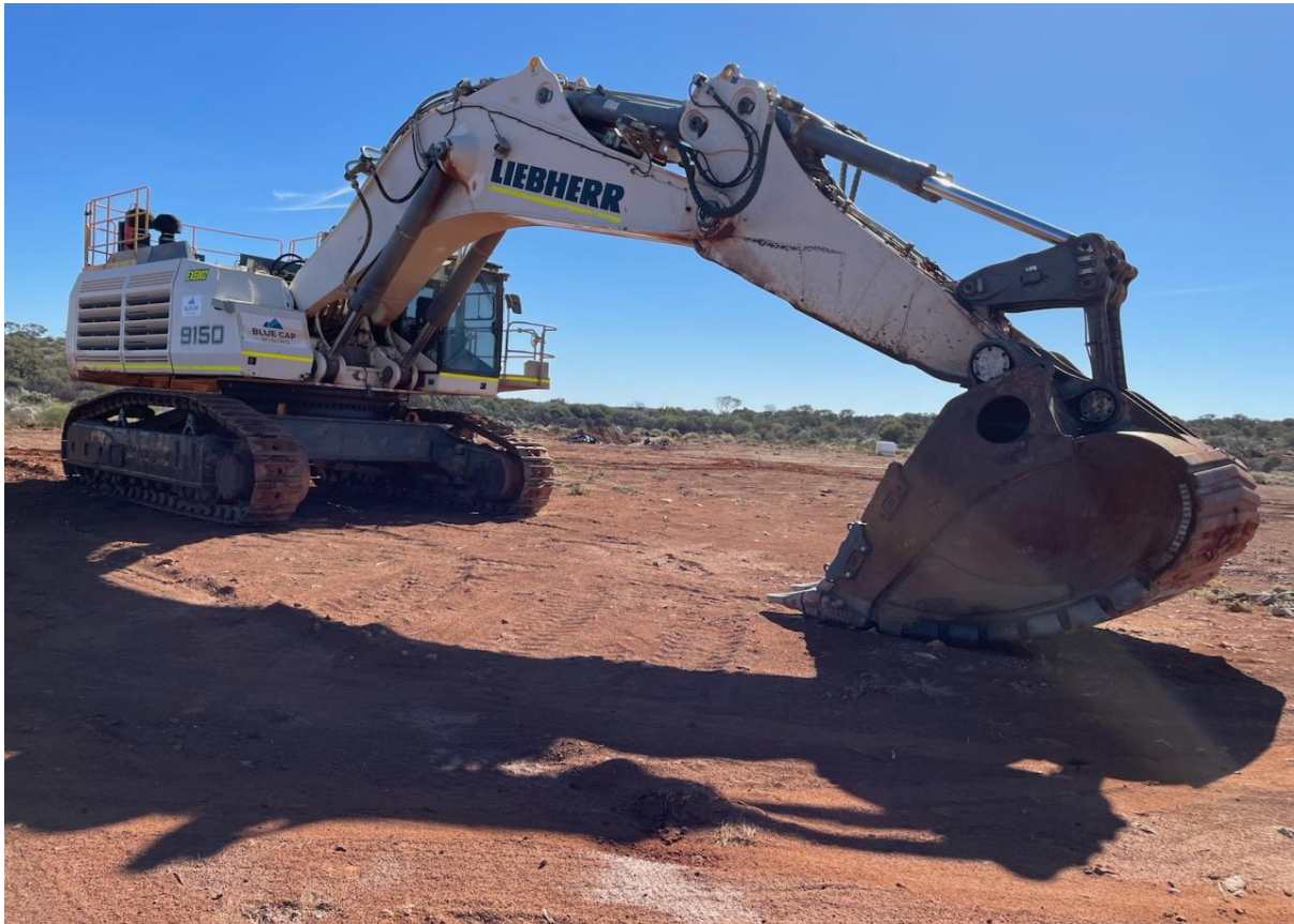
Plate 4 Liebherr 9150 Excavator on site
