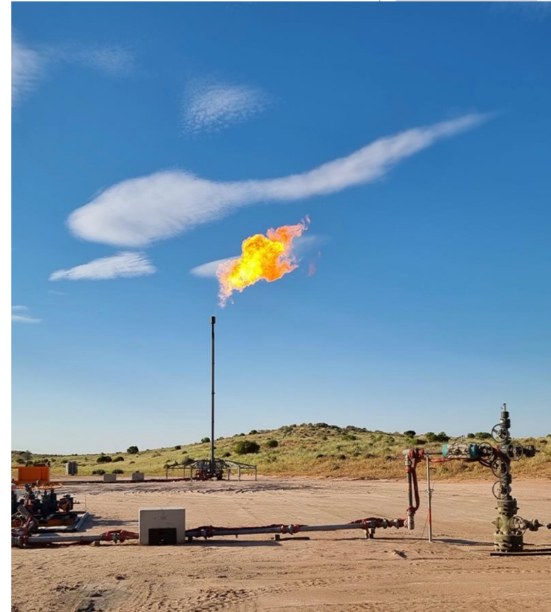
Figure 8: Gas flare from Kiwi-1 wellsite at 1.7 mmcf/d
