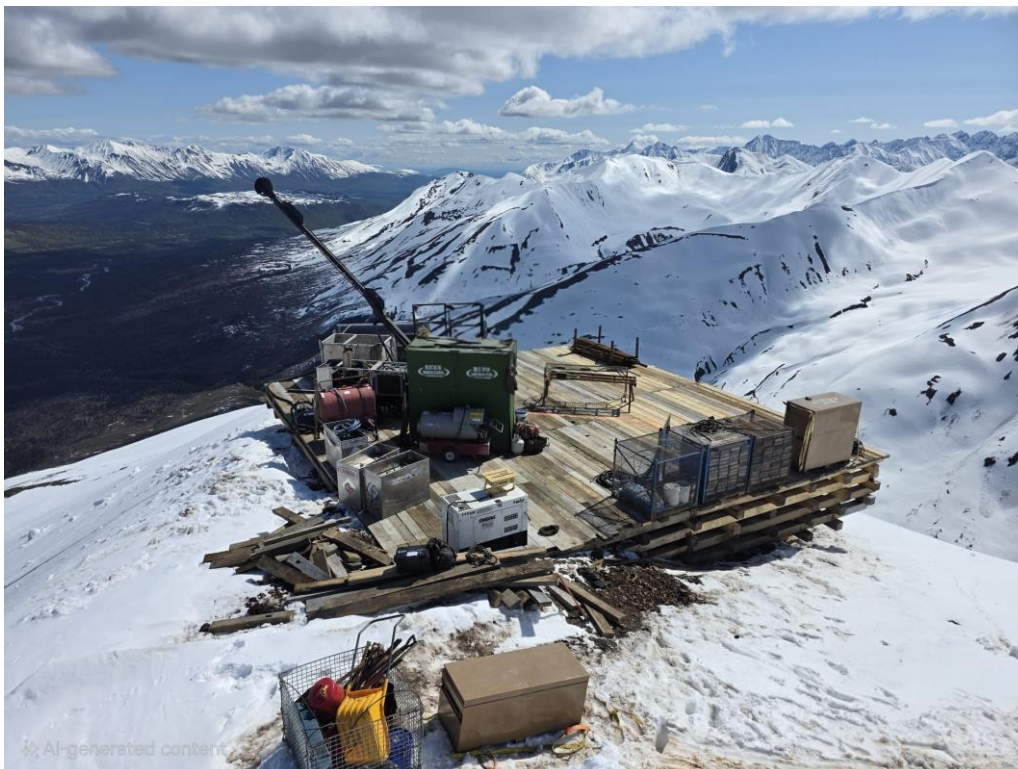
Figure 1. Drilling commenced at the newly built pad at Stibium
