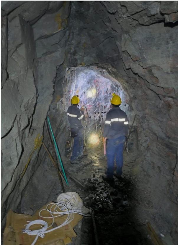
Development Drive Wired for Blasting
