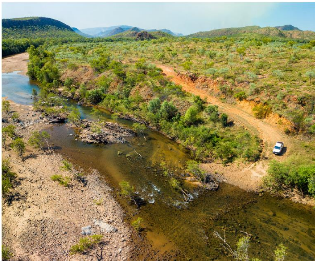
Figure 1: Photo of the existing historical Speewah access tracks at the Dunham River crossing
