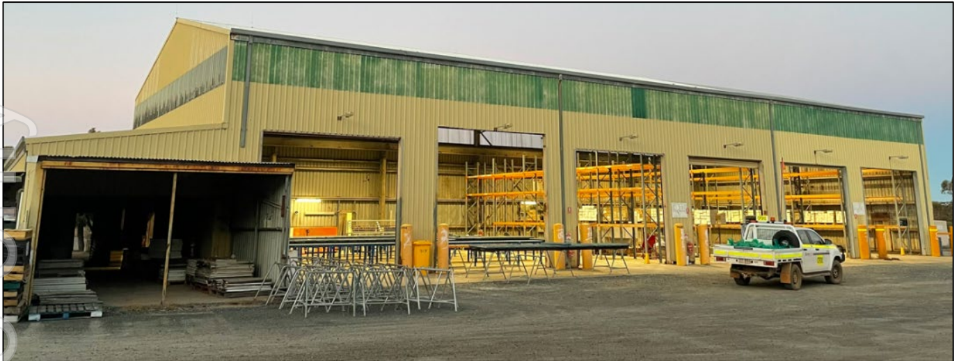
Figure 12: Foster Mine workshop
