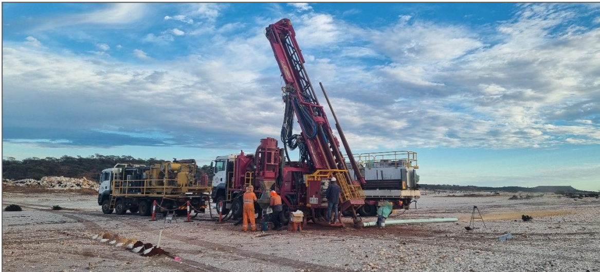
Figure 1. Cazaly commences their first RC hole to drill test Duke of York gold mineralisation.
