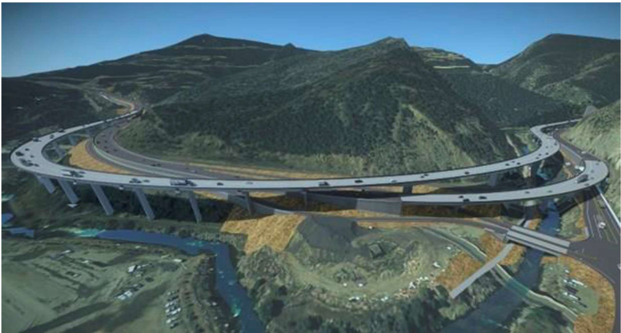
Figure 6. Model of I-70 Floyd Hill Project showing part of eight-mile section of I-70 Mountain Corridor
