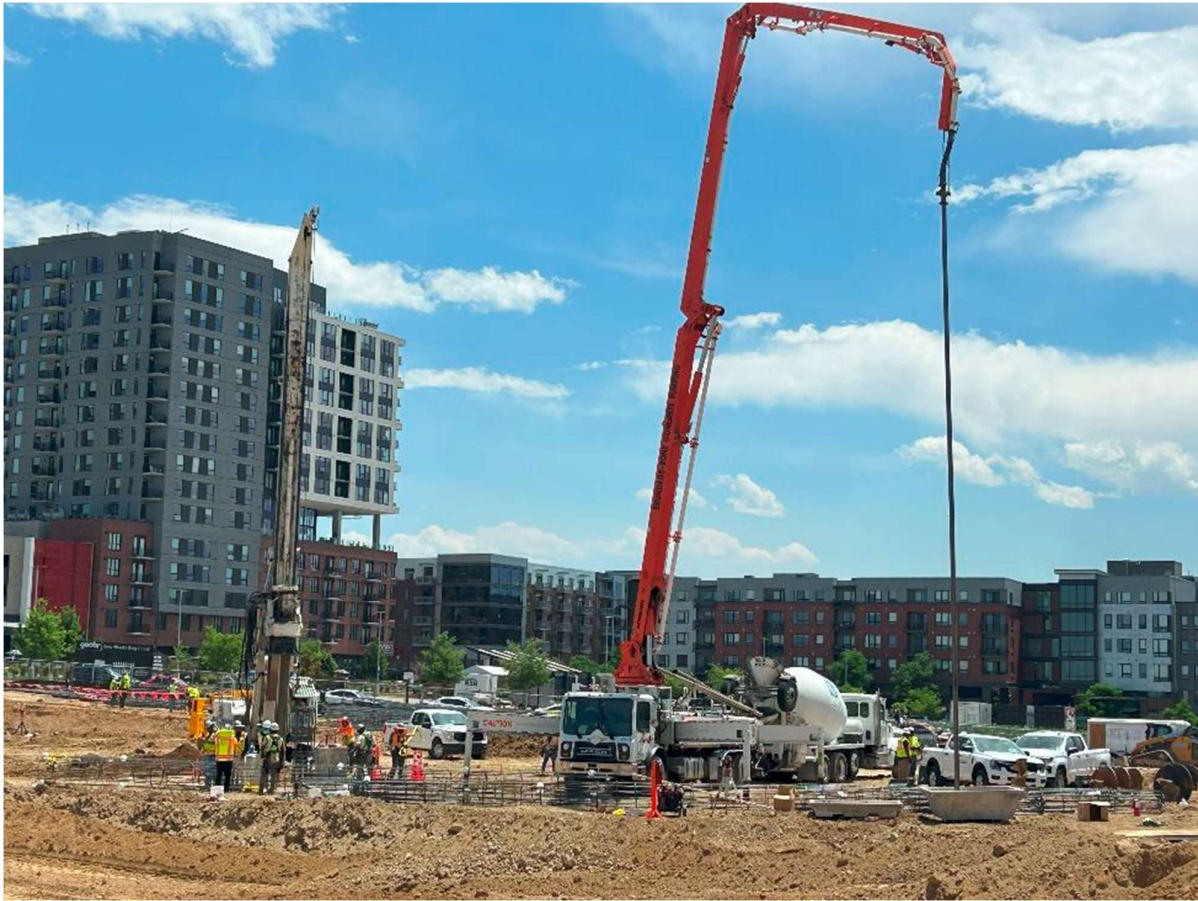
Figure 3. Pouring concrete for caissons
