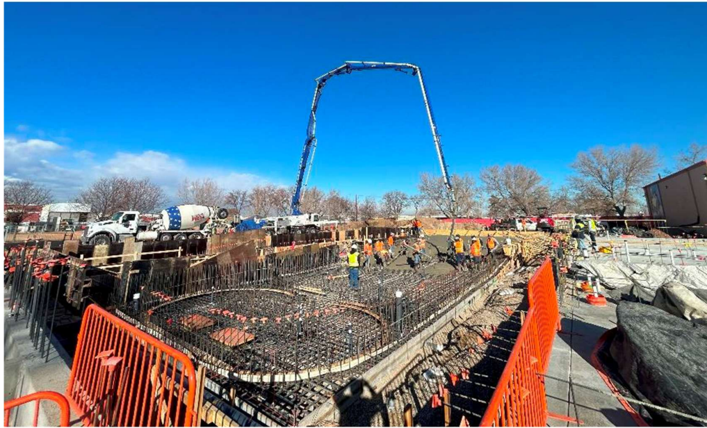
Figure 4. Pouring Concrete - Swansea Recreation Centre Swimming Pool
