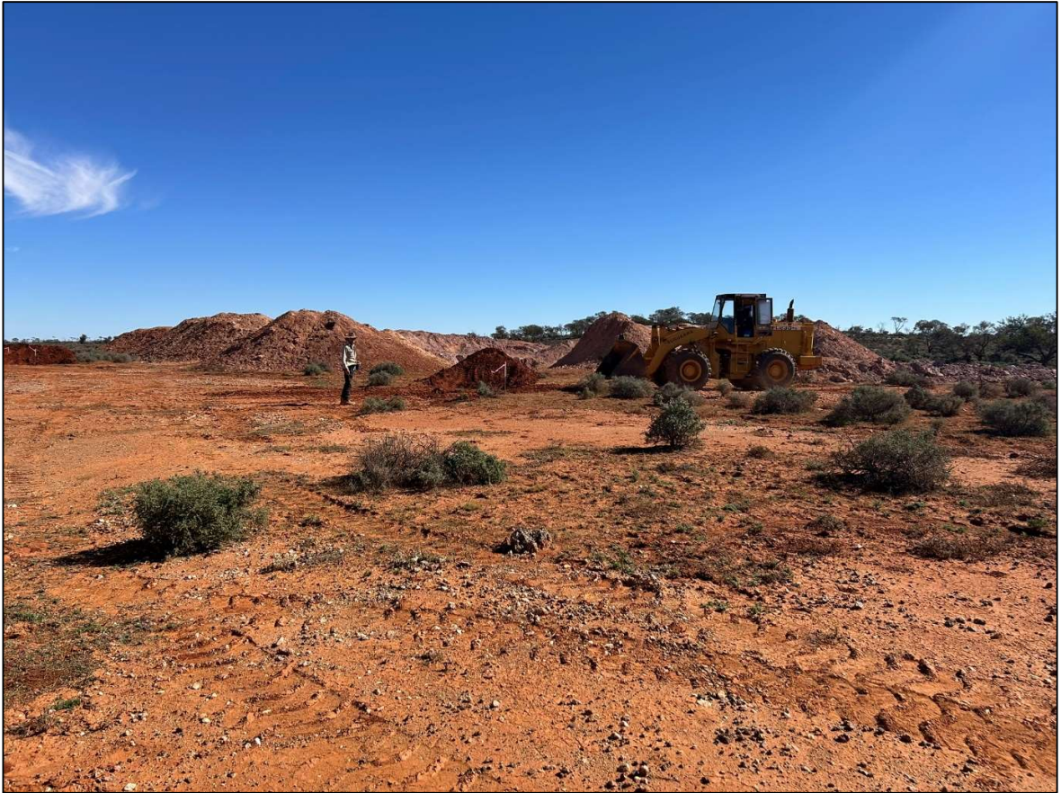
Figure 3: Drill site preparation, Killarney
