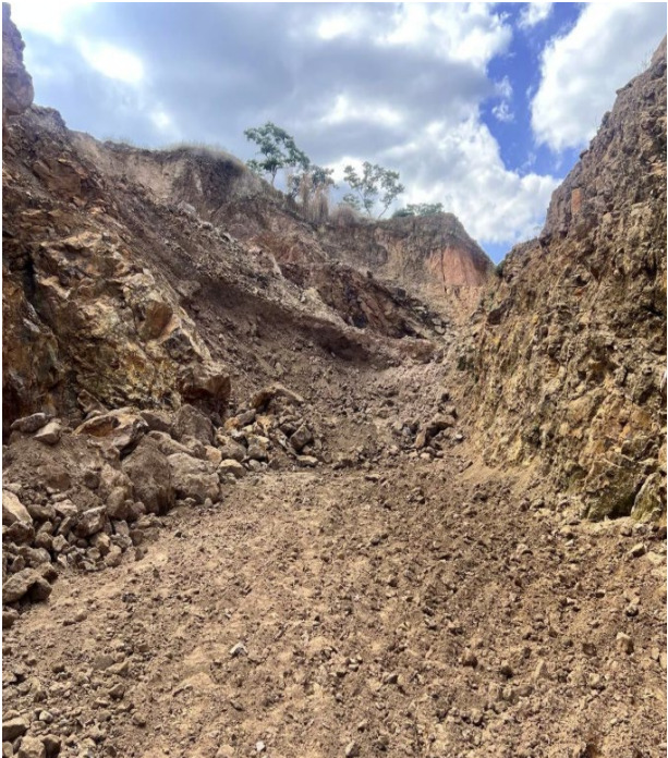
Image 1: Looking North East into the Sugarloaf pit
