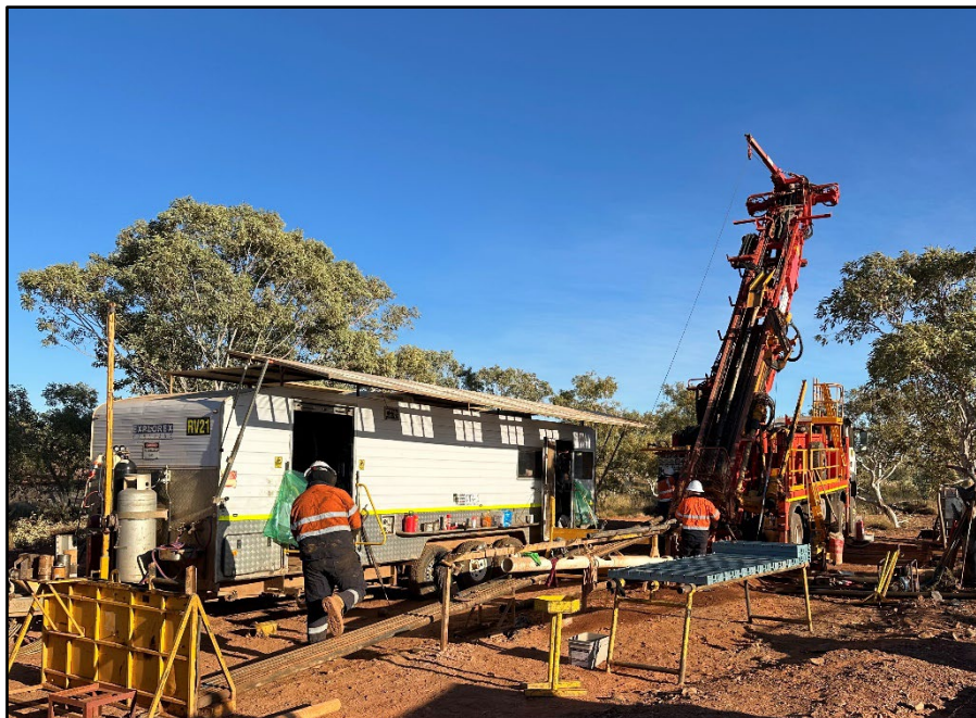
Photo 1: Geotechnical diamond drilling underway at the White Devil Gold Deposit
